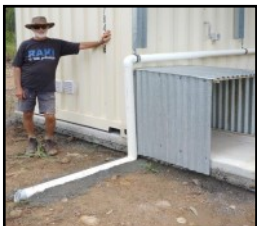
The finished project making sure that overflow water is discharged well away from the building.
