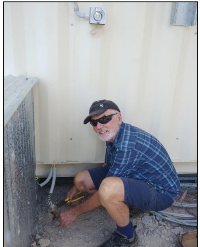
Ray VK2JU connecting the earthing wiring. Note the all weather 240 volt power inlet above.
