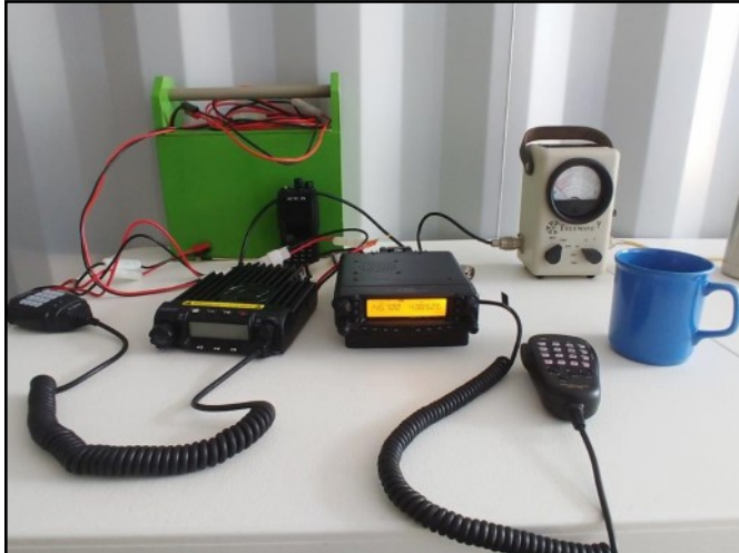
Antennas being tested with RF on air.
