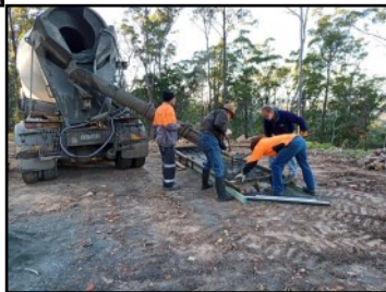
The concrete slabs poured, Ken Chainsaw shows how screeding should be done.
