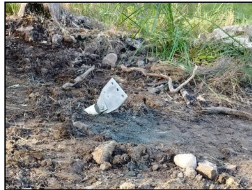
Mast Anchor block completed and backfilled North Guy
