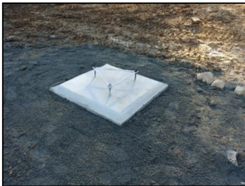
Mast foundation block completed
