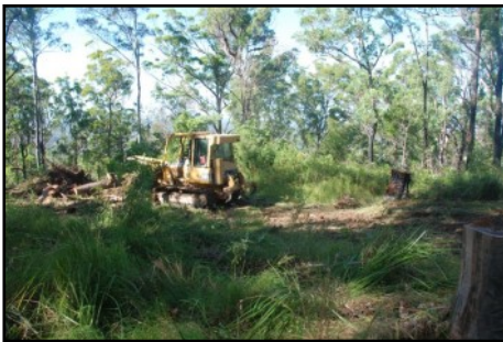
Starting work, clearing with the heavy equipment.
