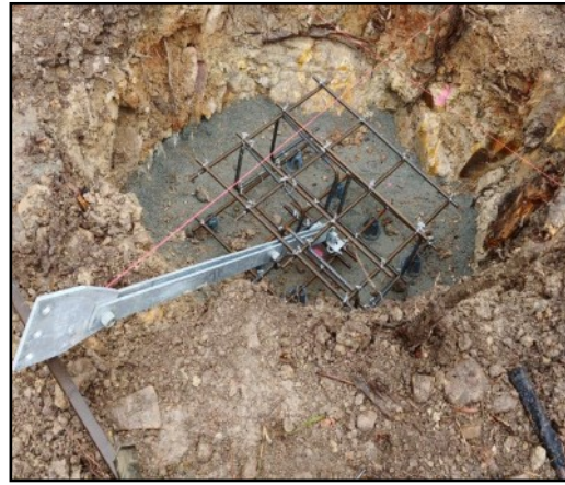
Mast North Guy Anchor block form-work.
