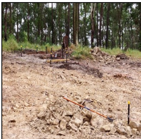
Mast Anchor block ready for concrete North Guy.
