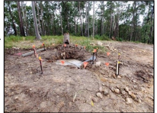
Mast Anchor block concrete North Guy
