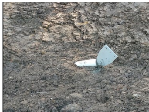
Mast Anchor block completed and back-filled South-West guy
