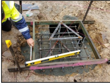
Mast Foundation block formwork
