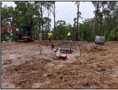
Positioning the site of the concrete block for the mast
