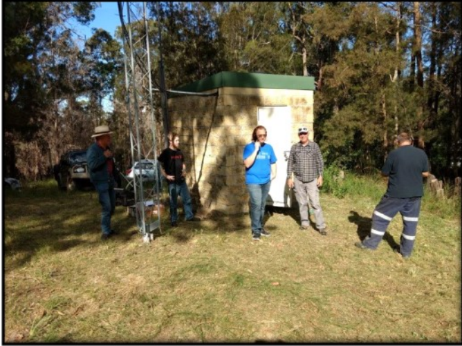
Part of the work crew on site.
