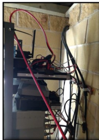
Above an impressive rack of repeater equipment.
