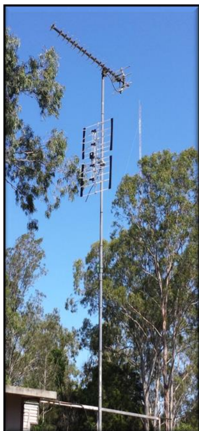
The New Matchmaster 02MM Antenna Mounted Beneath the Old Top Yagi
