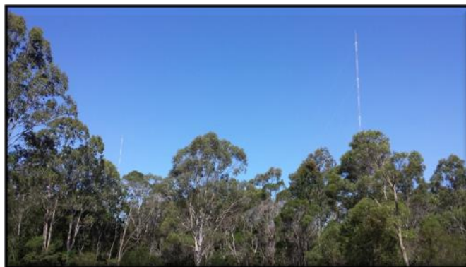
The Super Radio Network 531KHz AM Tx Phased Array Antenna Masts
