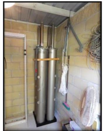
John Winchester VK2NJJ very kindly transported to the site the four coaxial filters that comprise the duplexer for the 6 metre repeater.
