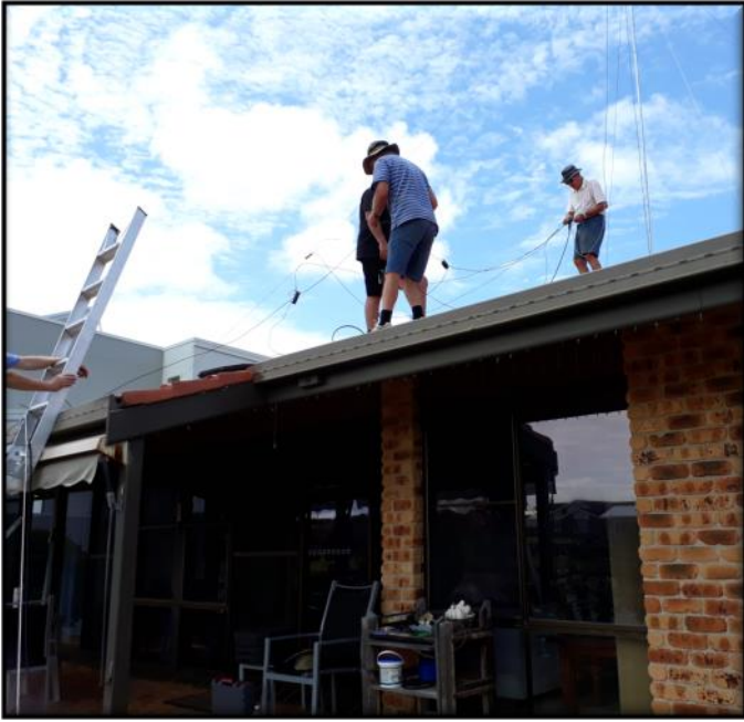
Antenna wires always have a life of their own and need careful sorting out. Rob VK2CRF, Lyle VK2SMI and Arthur VK2ATM laying out the traps and tuned lengths.
