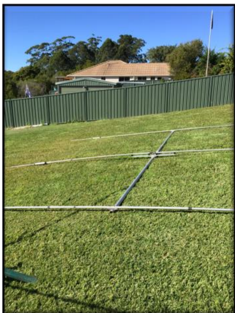
Antenna safely on the ground ready to be attached to the relocated mast. Fortunately Stuart VK2FSTU has a large back yard that enabled us to manoeuvre the 3 element beam which seemed considerably larger on the ground than in the air.
