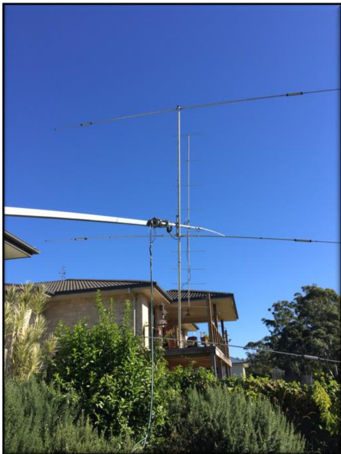
The mast tilted down ready for antennae removal.
