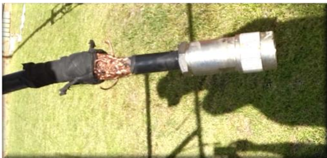
Antenna co-ax before fixing.
