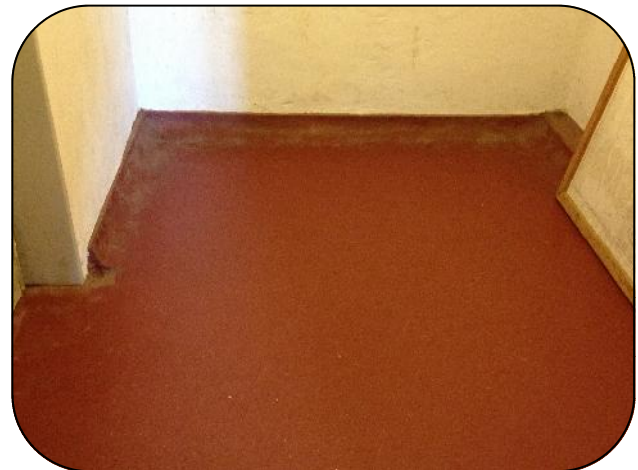
The battery room at the signal station. Note the bathtub like floor to help contain sulphuric acid spills.
