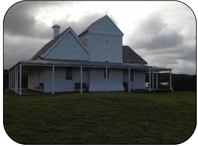
Cape Otway signal station restored today
