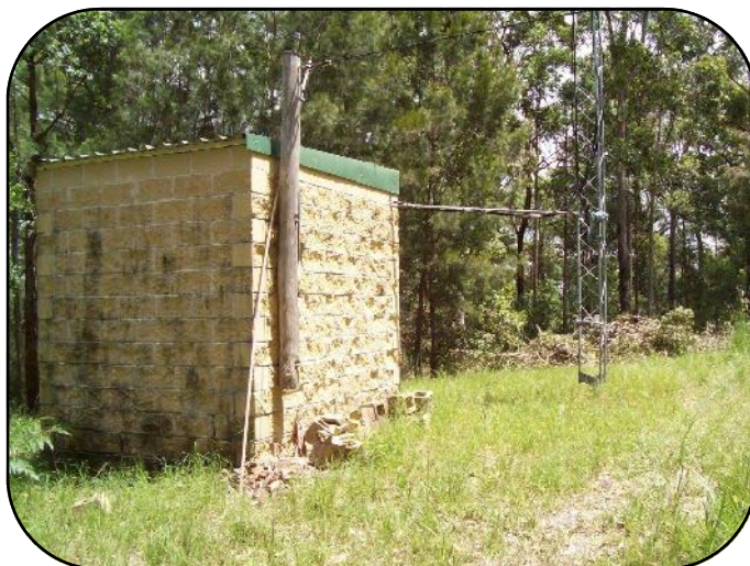
RCN repeater building Telegraph Point
