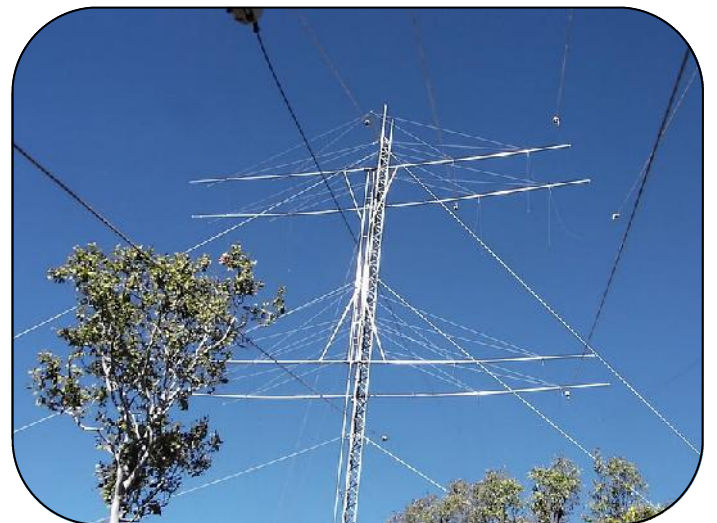
(Two views of the main towers being erected) (A close up of the South Eastern Asian antenna)
