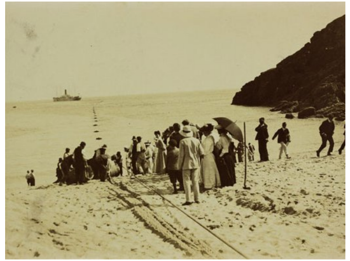
(Submarine cables being brought ashore at Porthcurno 1870)
