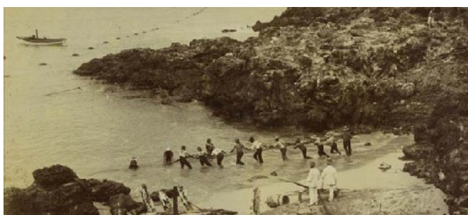
(Cables from the beach being carried to the telegraph station Cornwell).
