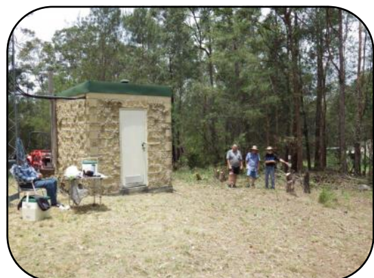
The ground is cleared to the repeater shack at Telegraph Point
