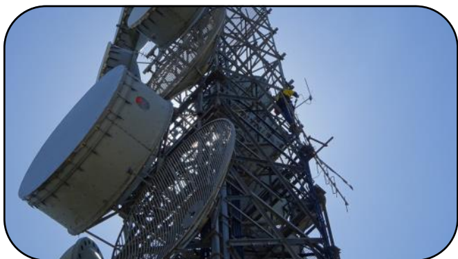
Communications antenna tower with club antennas mounted on right hand side of photograph.
