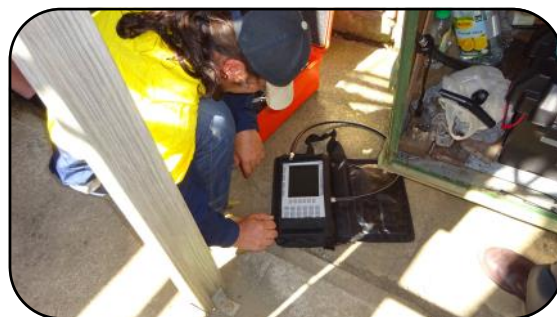
Frequency and return loss/time domain reflector (TDR) measurements
