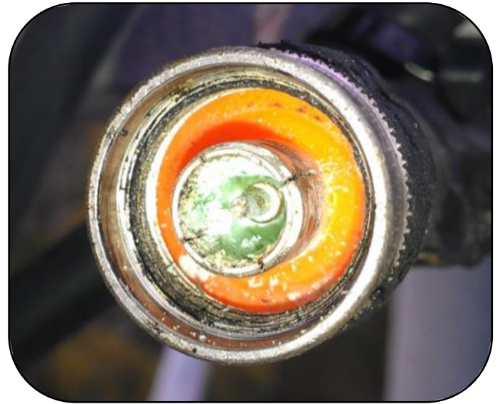
Note the amount of corrosion on the connector
