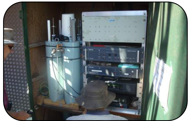
Arthur VK2ATM and Rob VKCRF work on the repeater.
