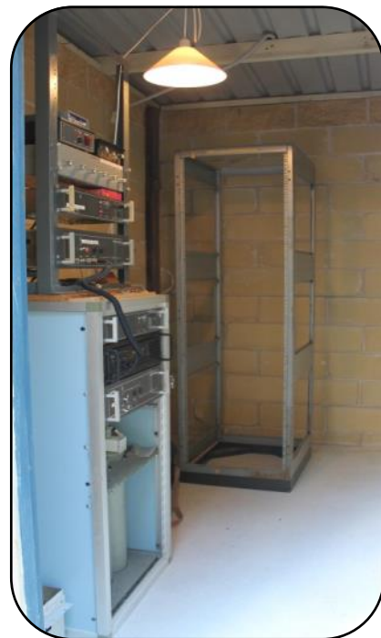
Rack in the Shack ready for 6 Metre Repeater
