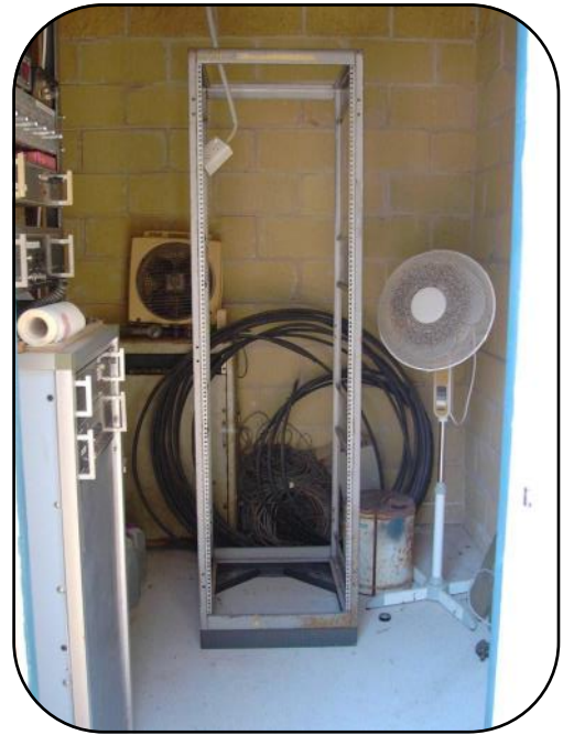
New rack to be installed
